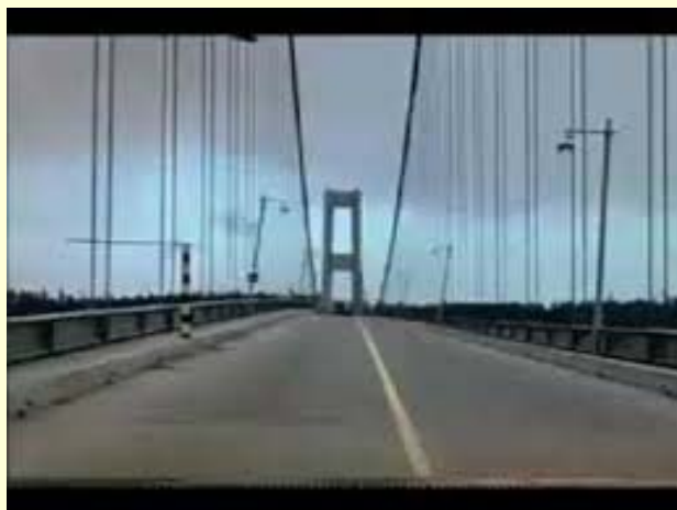
Tacoma bridge flutter instability (1940) [Wind speed: 40 mph]
